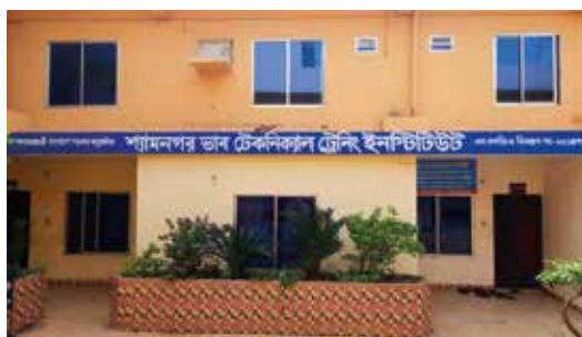
Shyamnagar VAB Technical Training Institute: VAB's maiden initiative for institutionalized skills development in the coastal area of Shyamnagar, Satkhira.
